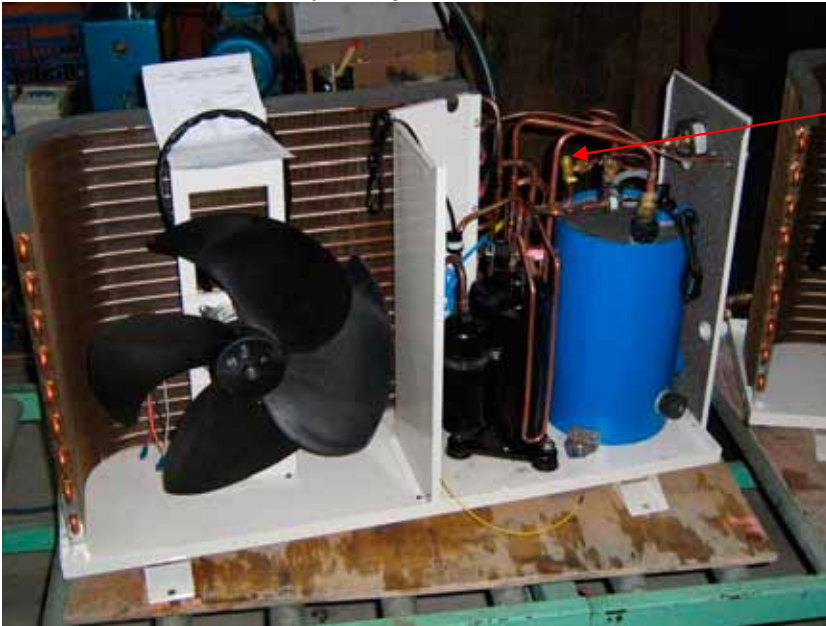
Figure 44: Manometer replacement.
