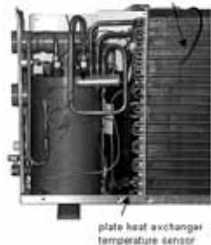
Figure 40: Plate heat exchanger temperature sensor.
