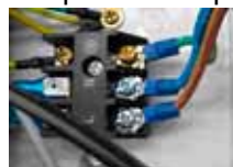
Figure 9: Mains connection terminals.
